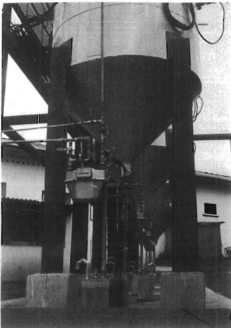
Fig.4. Pilot-scale metal storage bins with automatic interstitial nitrogen pressure maintenance device, gas meters and pressure relief valves.
